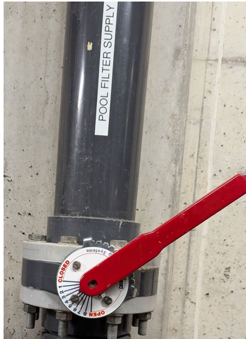
Figure 23: Pool Circulation Pump Control Valve
