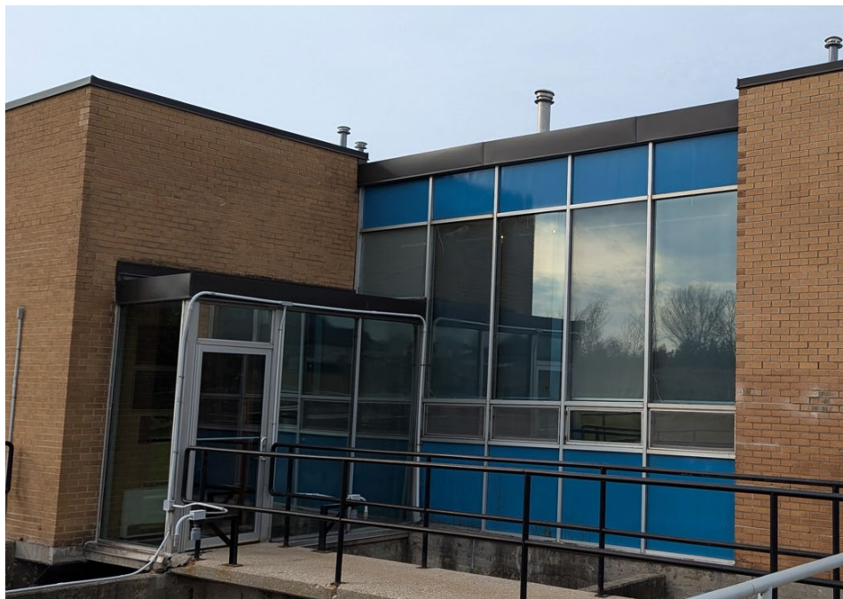
Figure 24: WWTP Control Room Curtain Wall
