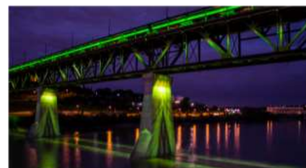
High-Level Bridge in Edmonton
