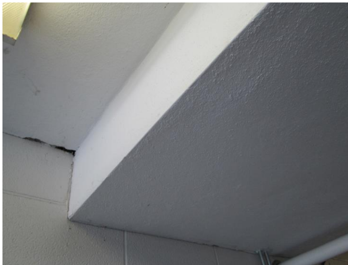
Photo 7: Textured Plaster (samples 19A-C) was sampled from the Foyer (Location 2) and was found to contain 1.4 – 1.6% Chrysotile asbestos.
