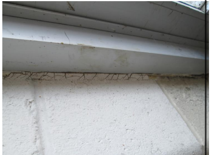
Photo 4: Yellow Door Caulking (samples 5A-C) was sampled from Entryway #2 (Location 9) and was found to contain 1.2% Chrysotile asbestos.
