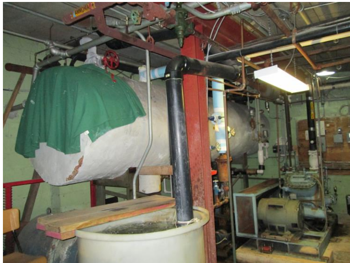
Photo 3: Mechanical Parging (Parged Chiller) (samples 7A-C) was sampled from the Mechanical room (Location 13) and was found to contain 60% Chrysotile asbestos.
