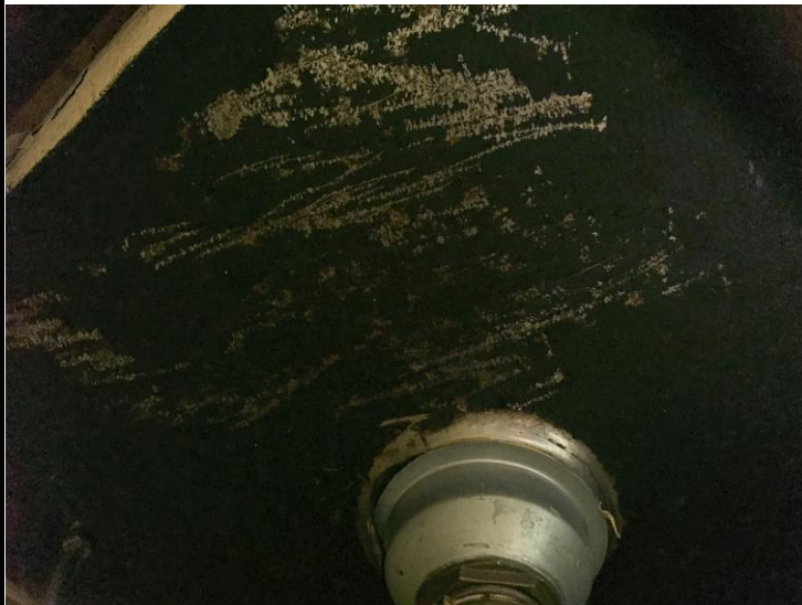
Photo 10: Sink Undercoat (samples 4A-C, 2019) was sampled from the Concession Area (Location 46) and was found to contain 8% Chrysotile asbestos.
