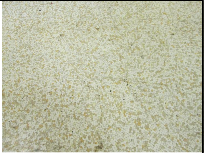
Photo 6: Yellow Chicklet vinyl sheet flooring (samples 18A-C) was sampled from the Concession area (Location 46) and was found to contain 20% Chrysotile asbestos.
