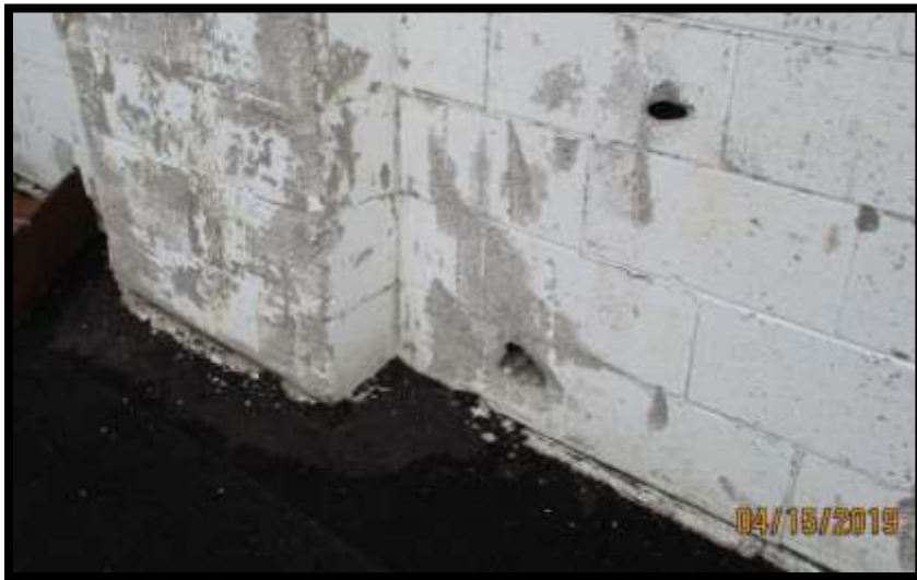
Abrasion and puncture of blocks on south wall
