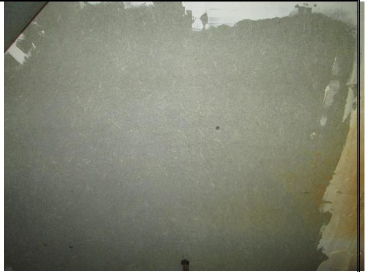
Photo 2: Transite ceiling panels (Samples 1A-C, 2019) sampled from the furnace room (Location 4) were found to contain 10% Chrysotile asbestos.
