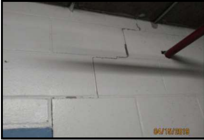
Pattern crack in change room partition
