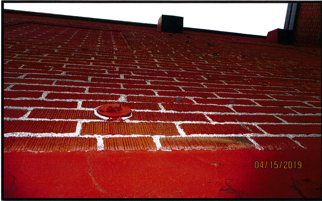
Bulging north wall, showing tie-back bolts.
