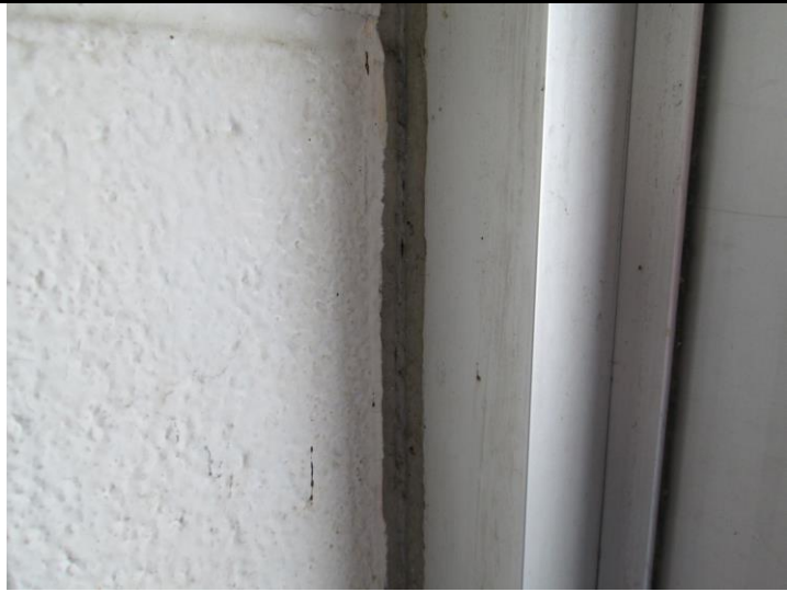
Photo 1: Grey Door Caulking (samples 1A-C) sampled from the Entryway (Location 1) was found to contain 1.3% Chrysotile asbestos.
