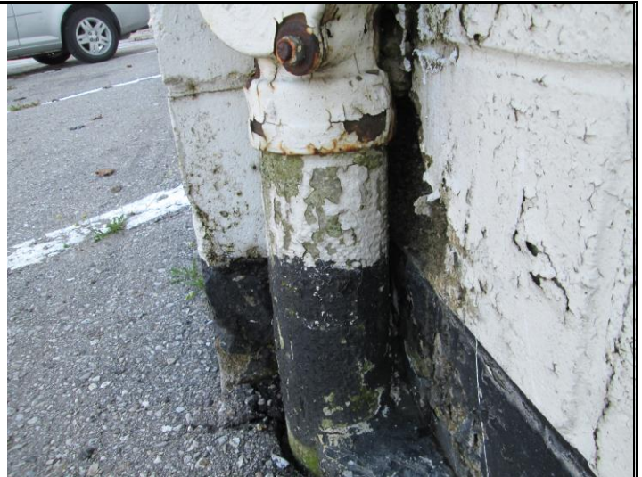
Photo 10: Transite Drain Pipe (samples 2A-C, 2019) was sampled from the exterior of the building was found to contain 5% Chrysotile and 5% Crocidolite asbestos.
