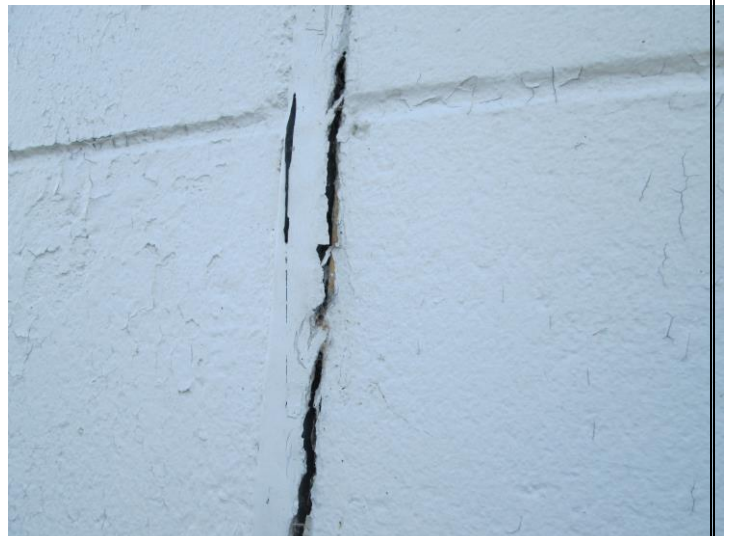
Photo 8: Expansion Joint Caulking (samples 20A-C) was sampled from the exterior of the building and was found to contain 1.2% Chrysotile asbestos.
