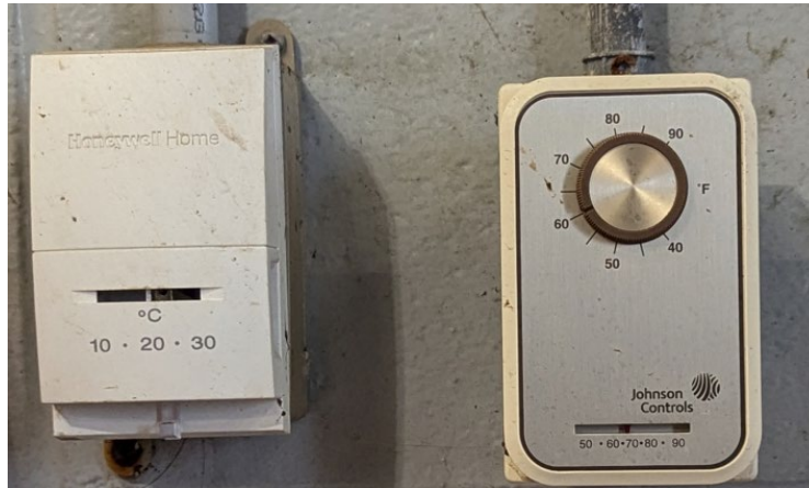
Figure 20: WWTP Existing HVAC Controls
